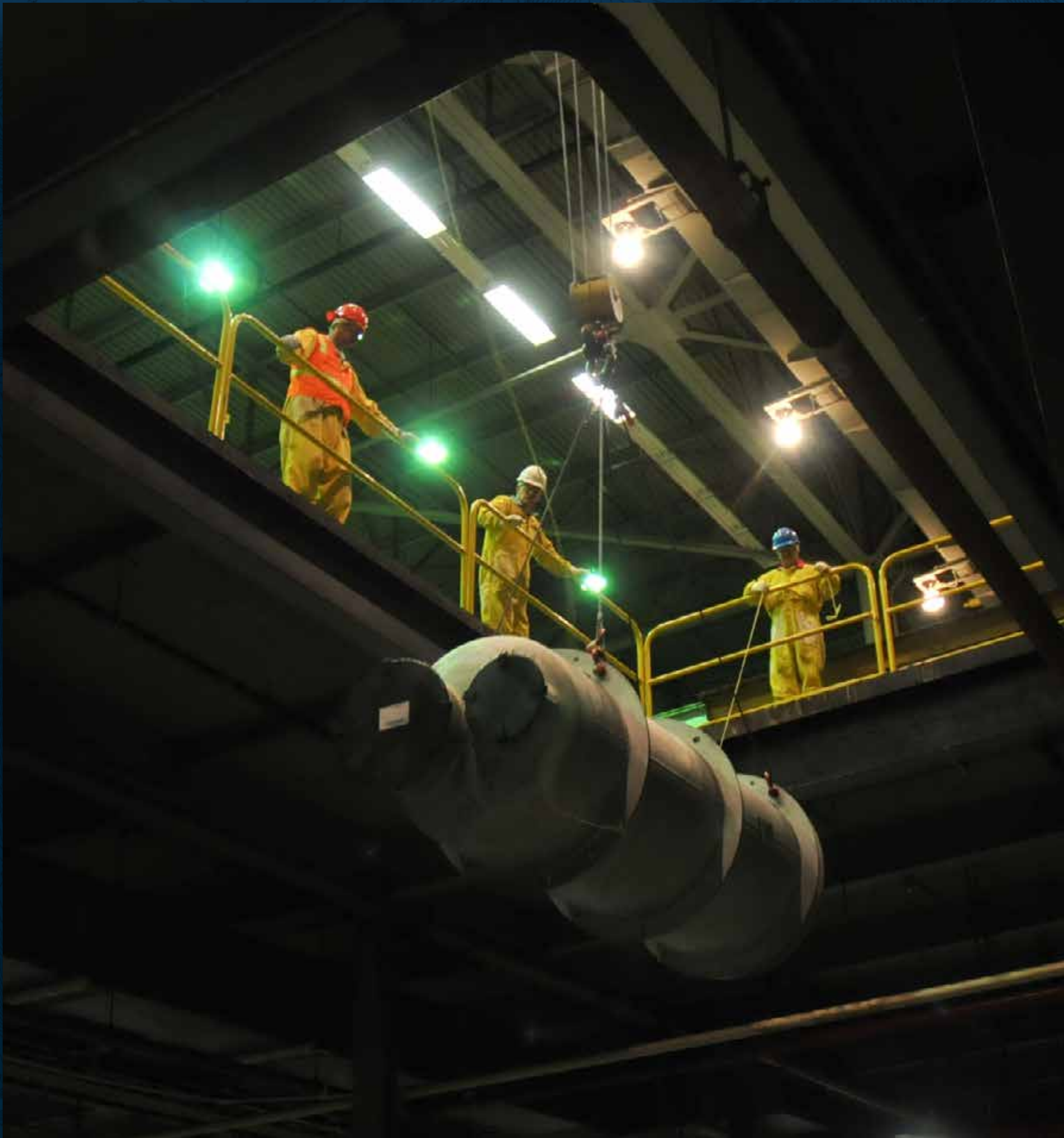
Converter lowered in preparation for disposal
