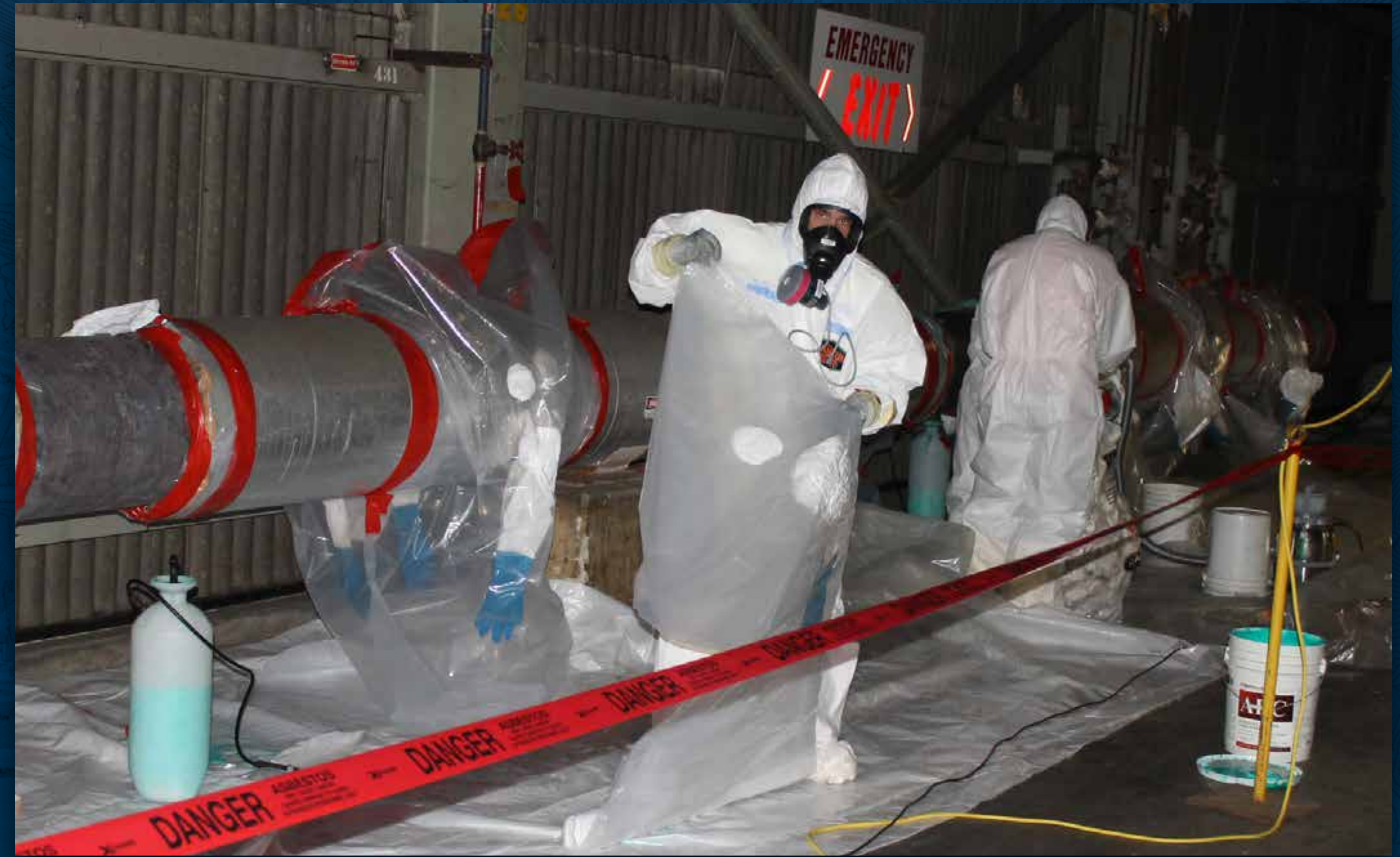
Bulk asbestos removal completed Sept. 30, 2019
