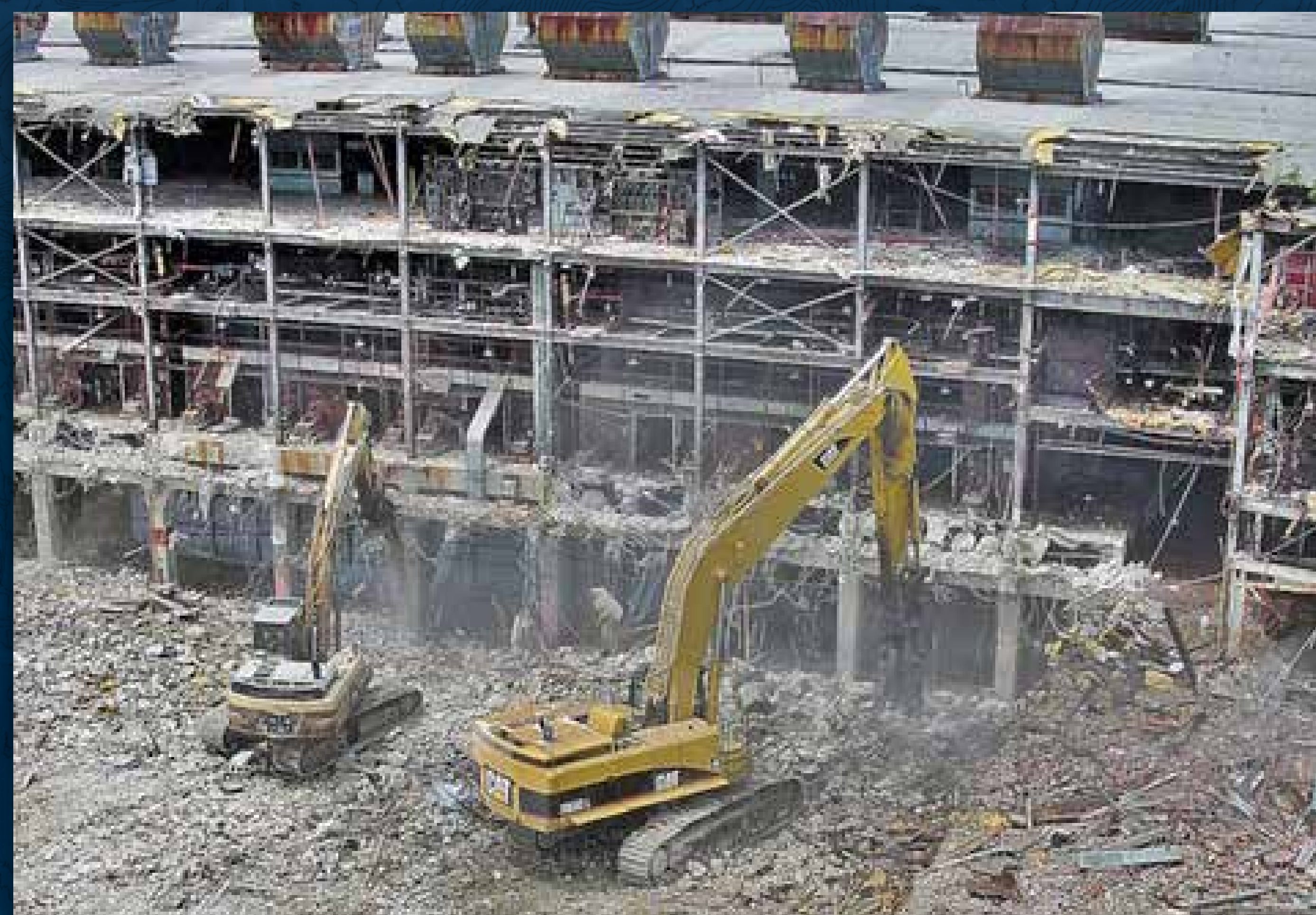
Demolition in Oak Ridge, TN
